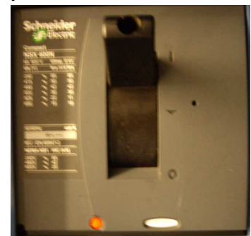
Figure 1 - 400amp circuit breaker shown in the on position
