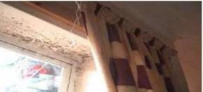
Rising damp or damp coming into the property (for example leaking gutters) coming into the property will appear as a damp stained patch, and in some cases the plaster can be coming away from the wall. Another sign is a white powder or salt coming to the surface of the wall. If the property has just had a damp proof course, salt on the walls can be due to the wall drying out.
