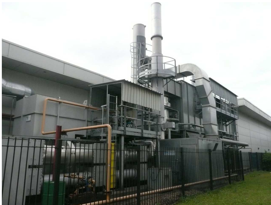
General view of RTO's and exhaust stacks – the Donau Carbon RTO is on the right
