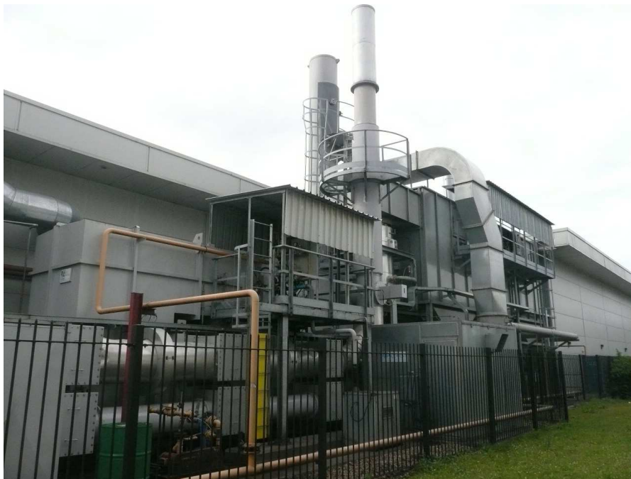
General view of RTO's and exhaust stacks – the Siri is on the left and Donau Carbon RTO on the right
