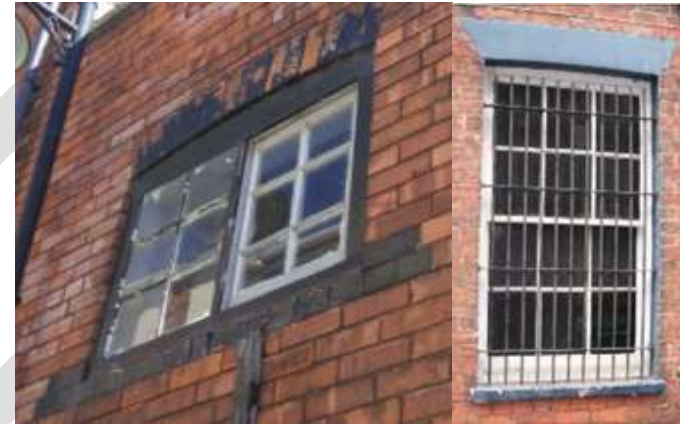
Left) 6/6 Yorkshire sliding sash on Wardall Street. (Right) Vertical box sash 6/6 on New Road.
