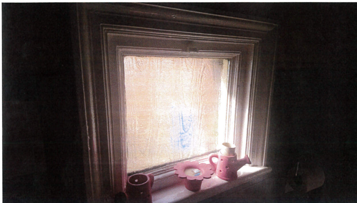
Photo 6- Original sash window- internal architrave detail
