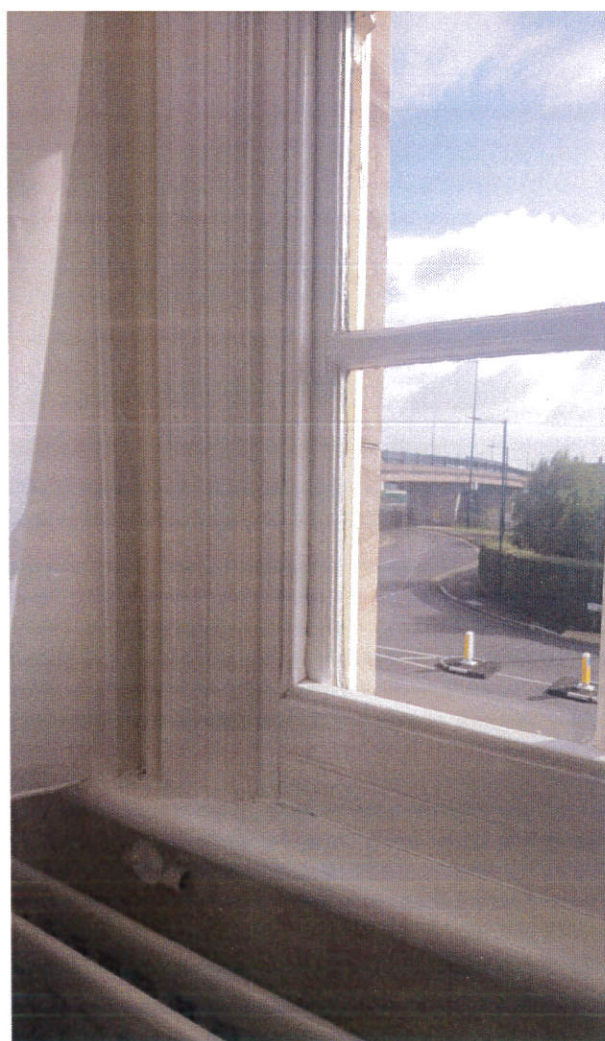
Photo 6- Original sash window- internal architrave detail
