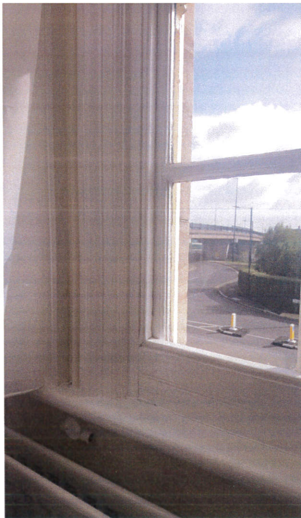
Photo 6- Original sash window- internal architrave detail
