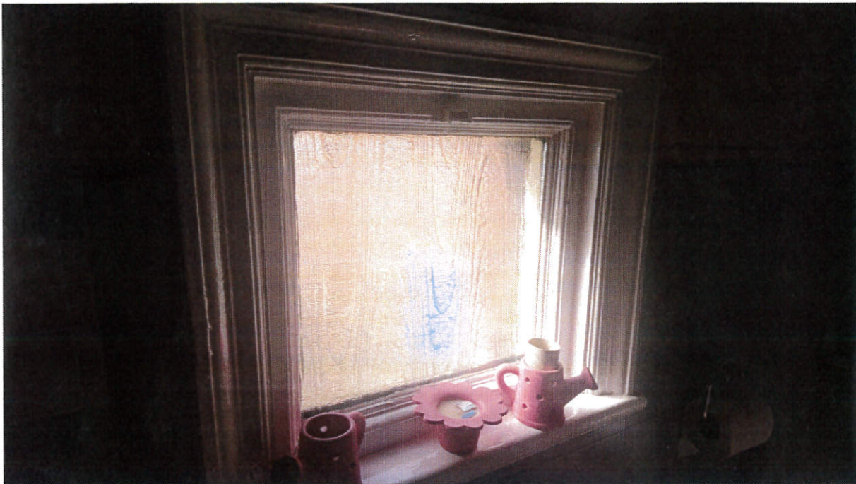
Photo 6- Original sash window- internal architrave detail
