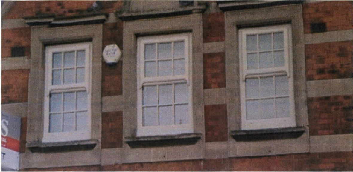
Photo 1- First floor showing 3 double glazed windows to front elevation
