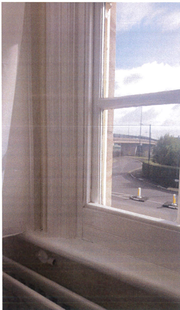
Photo 6- Original sash window- internal architrave detail
