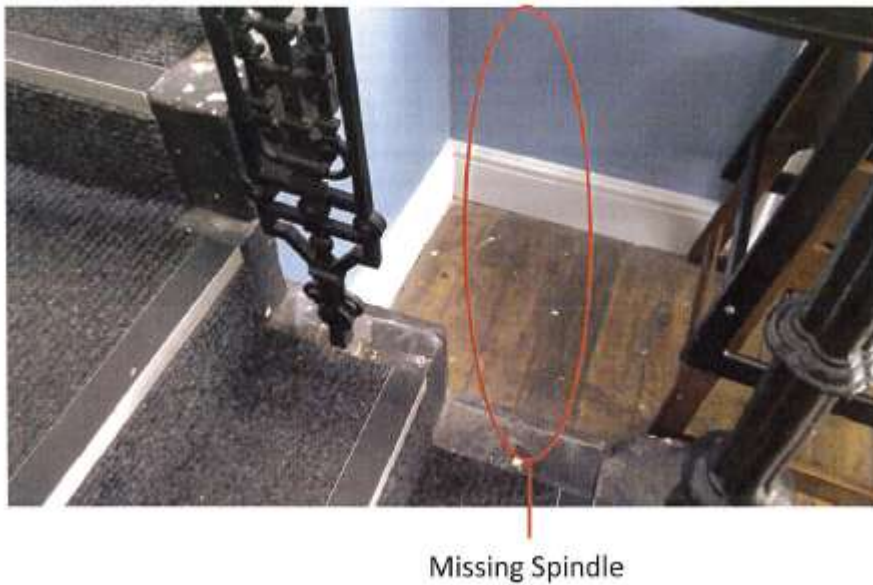
Photo 9 – Showing orientation of spindles
