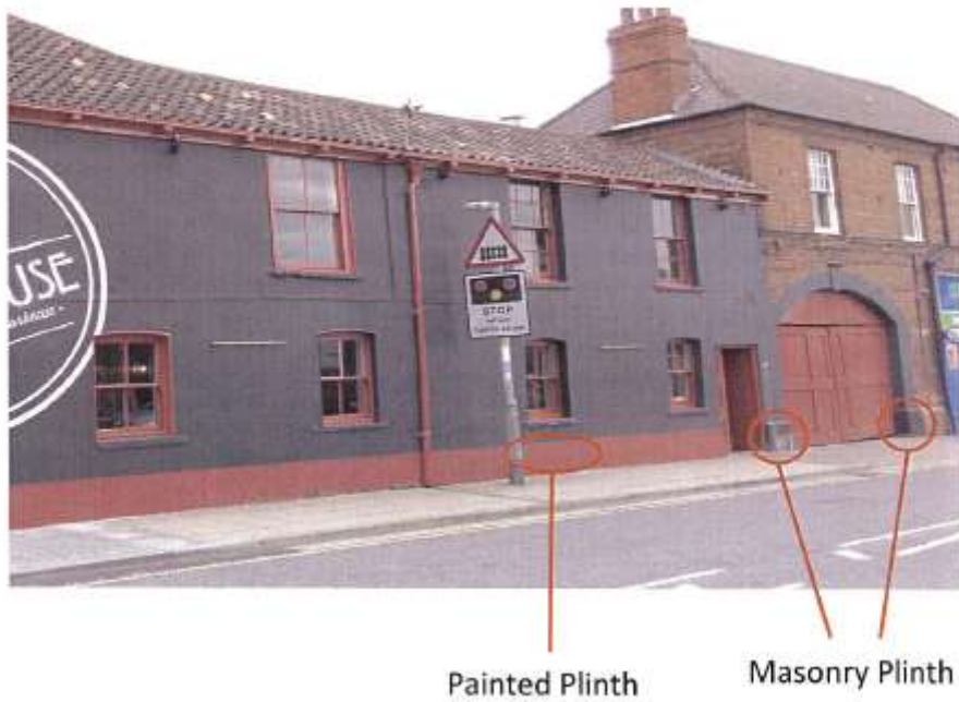
Photo 7 – Showing Wellowgate elevation including masonry plinth and painted plinth
