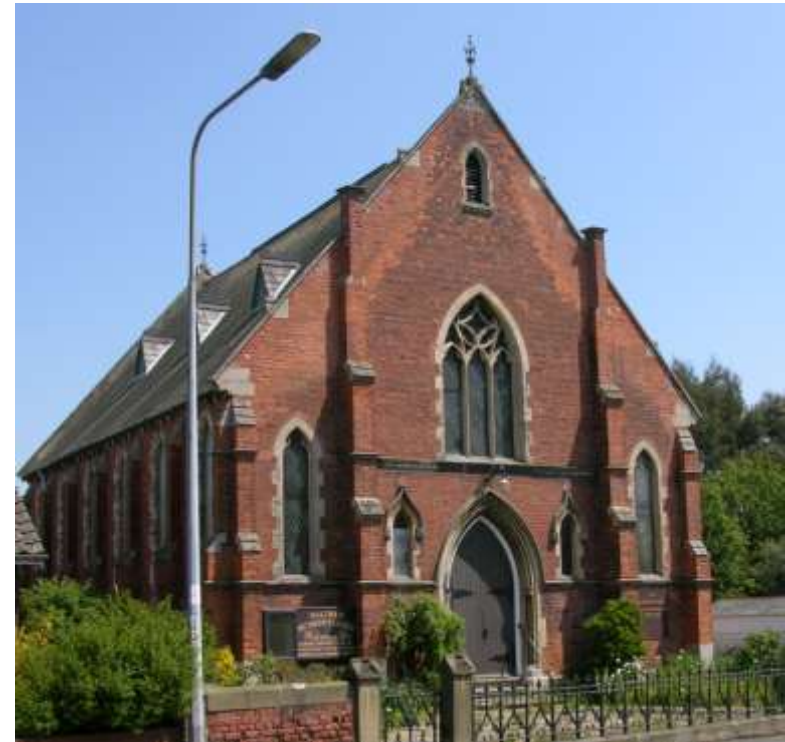
Waltham Methodist Chapel, Cheapside. Gothic style. Red brick with ashlar dressings, buttresses, slate roof with triangular dormers. High quality cast iron railings and gate in a lace like pattern
