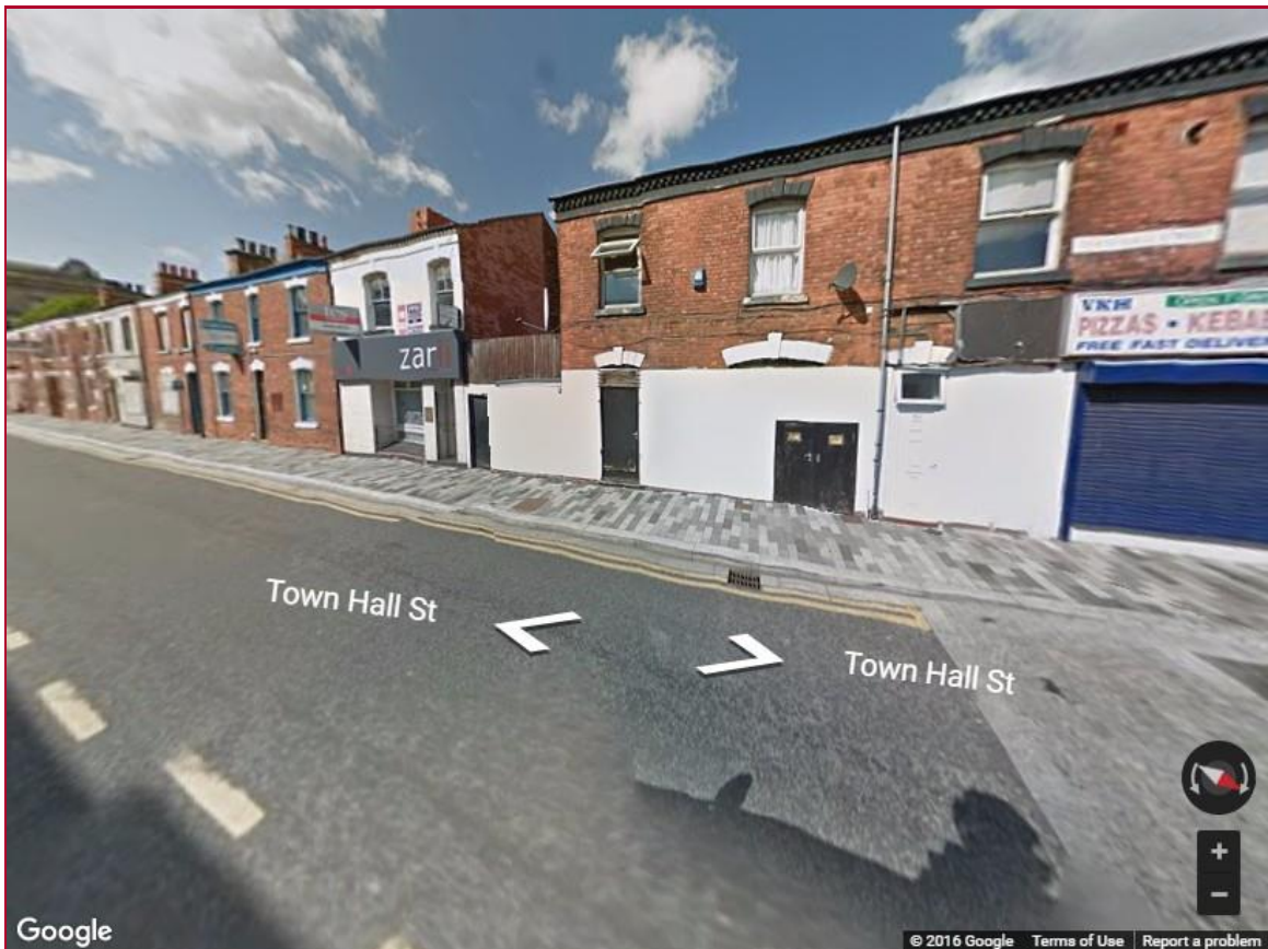
Figure A3. 5 – Townhall Street - ‘R52’ and ‘R53’
