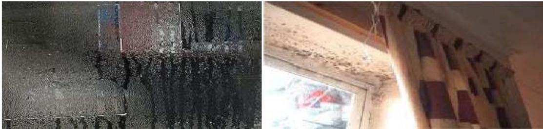
Rising damp or damp coming into the property (for example leaking gutters) coming into the property will appear as a damp stained patch, and in some cases the plaster can be coming away from the wall. Another sign is a white powder or salt coming to the surface of the wall. If the property has just had a damp proof course, salt on the walls can be due to the wall drying out.
