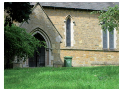
Church at East Ravendale
