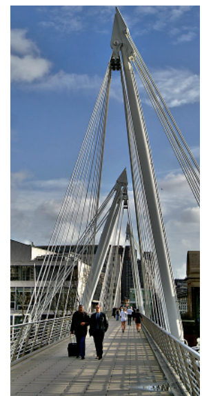
Example of a good pedestrian footbridge
