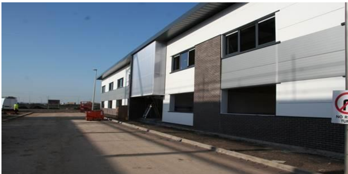
CATCH3 Training Facility, Stallingborough
