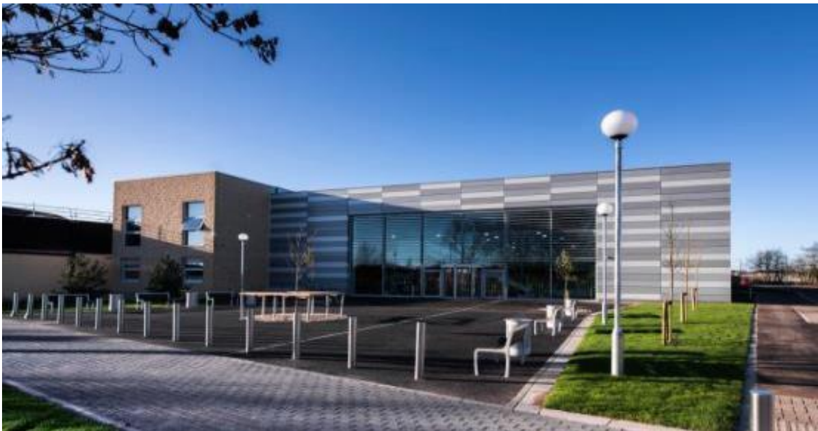
Grimsby Leisure Centre - extension and new pool.
