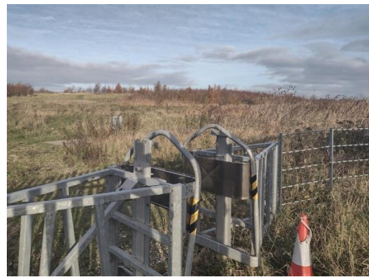
Photo 16 Entrance to Macaulay Lane Country Park
