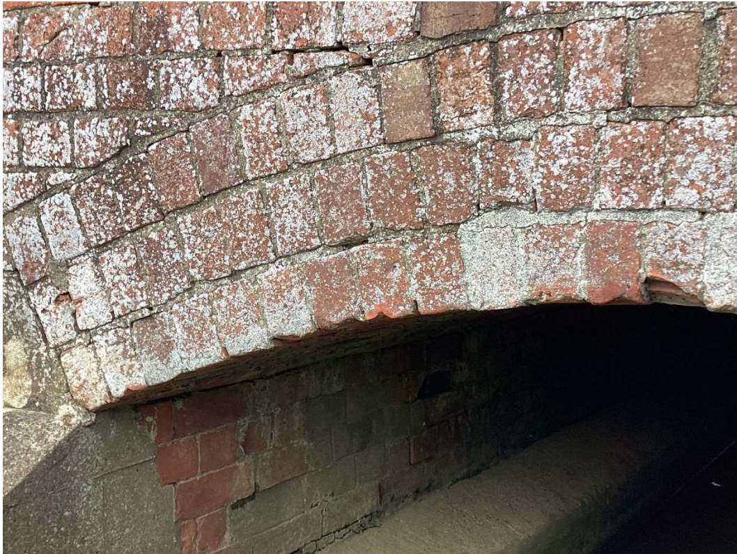
Waithe Lane Bridge Showing Missing Mortar and Poor Brick Structure Under Bridge
