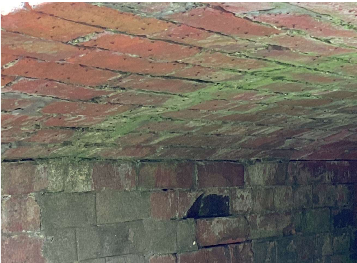
Under Waithe Lane Bridge Roof of Bridge and Side Wall Showing Missing Mortar Miscellaneous Use of Bricks Very Poor Condition
