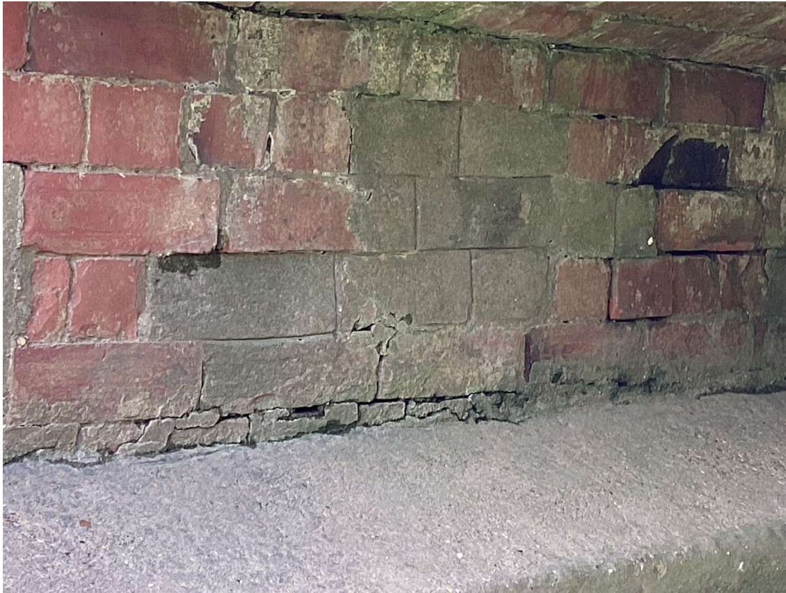
Under Waithe Lane Bridge Showing Poor Miscellaneous Use of Bricks Many Cracks and Missing Mortar Poor Condition
