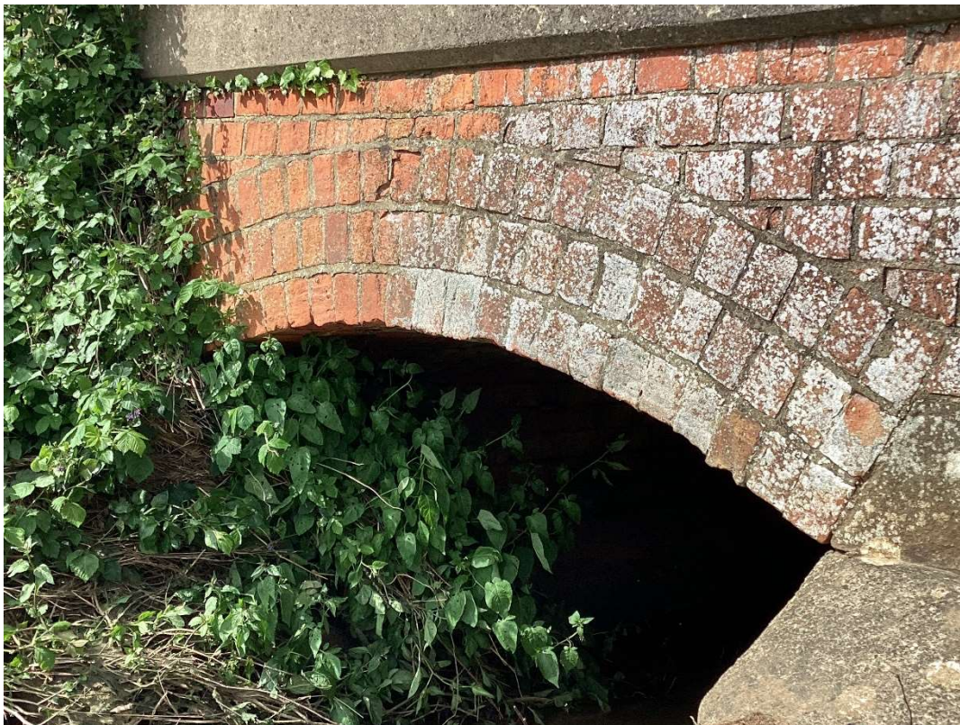
Waithe Beck Bridge Showing Crack Down Centre of Arch
