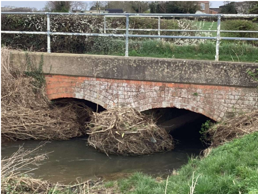
Waithe Lane Brigsley Beck Showing Poor Brickwork
