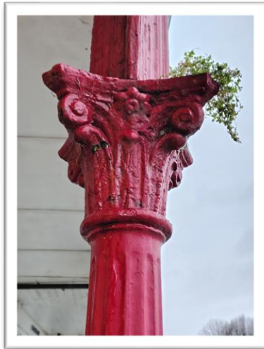
Examples of rust spotting and vegetation growth
