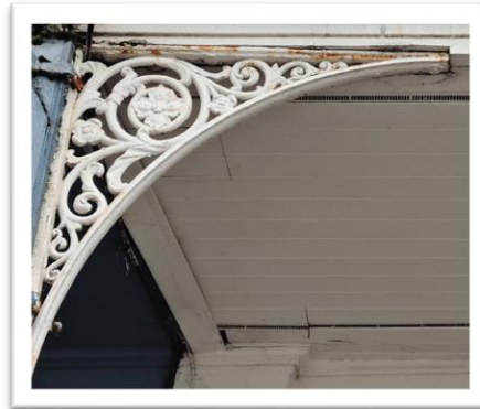
Examples of rust spotting and vegetation growth
