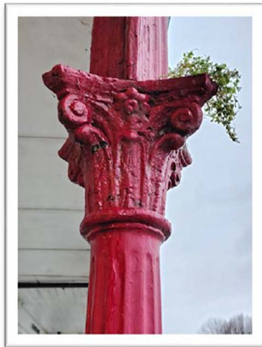
Examples of rust spotting and vegetation growth
