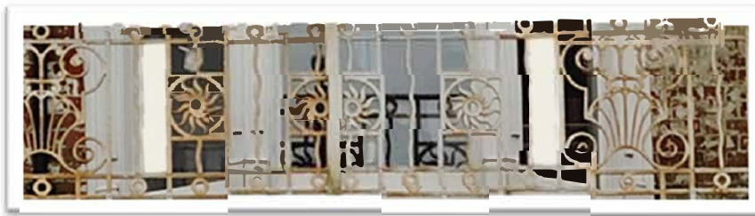
Example of cast iron which has been stripped back to the metal and not had the correct propriety coatings applied for a marine environment
