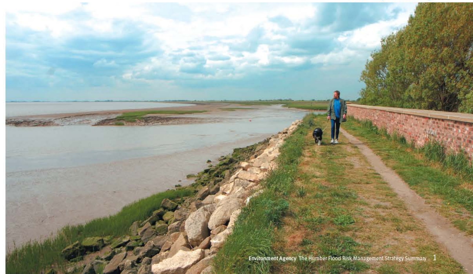
Flood defence at Brough
