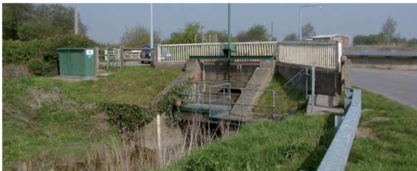
↑ Winterton Beck Outfall
