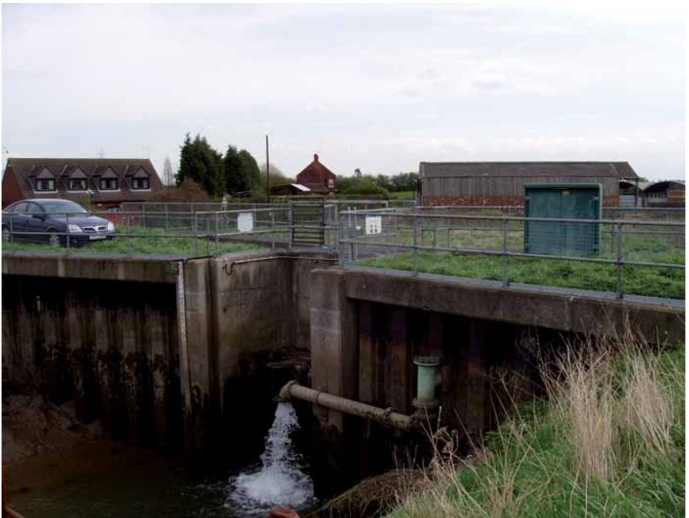
↑ Barrow Haven Sluice
