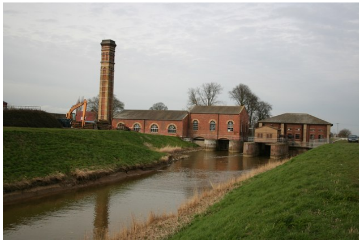
Lade Bank Pumping Station ©Richard Croft
