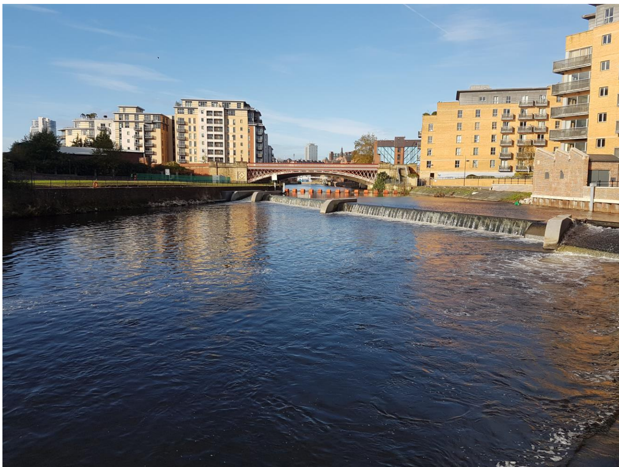
Figure 4: Leeds Flood Alleviation Scheme 1
