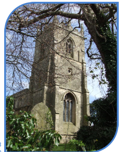
Footpath 13 Immingham Church
