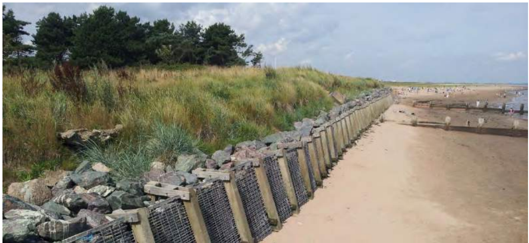
Photograph 2.2 – Recently replaced gabions at toe of dunes
