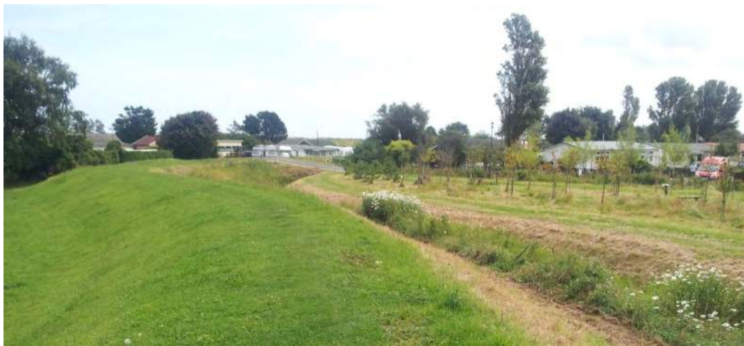
Photograph 2.4 – Primary flood defence embankment
