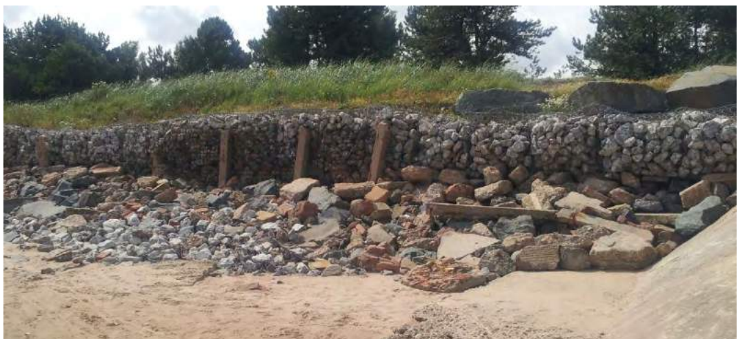
Photograph 2.3 – Old gabions in poor condition
