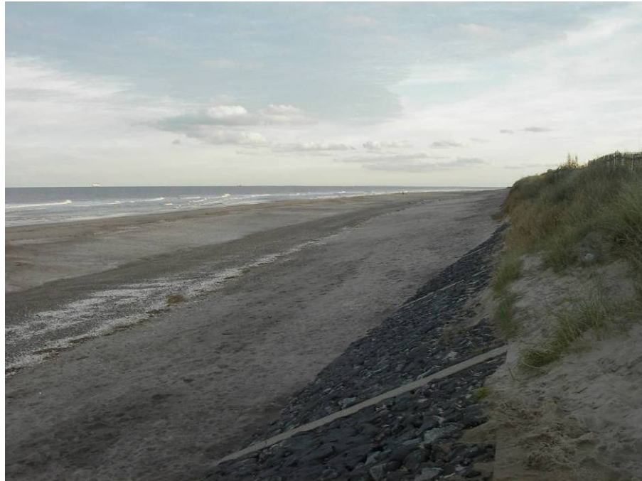
Figure 4.7: Armoured dune at Chapel Six Marshes
