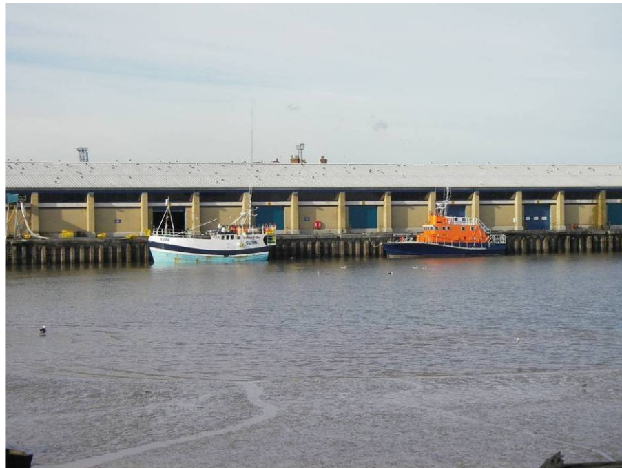
Figure 4.9: Sheet-piled quay within Grimsby's docks
