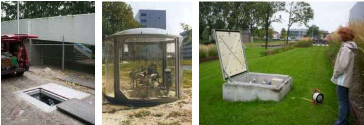
Figure 3-2: Example images of a housing for a single borehole for a WSHP system 6
